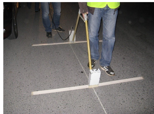
Investigating with GPR
