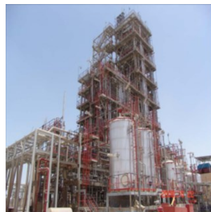
PVM demonstration plant with capacity of 1 ton/day methanol
