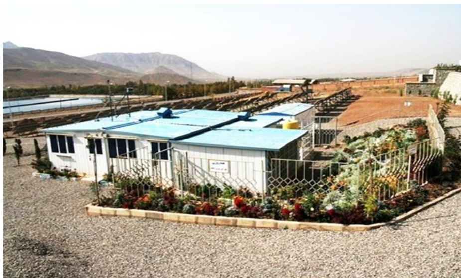
Taleghan Renewable Energy Park: Center for H2 & FC technology demonstration and other types of renewable energy
