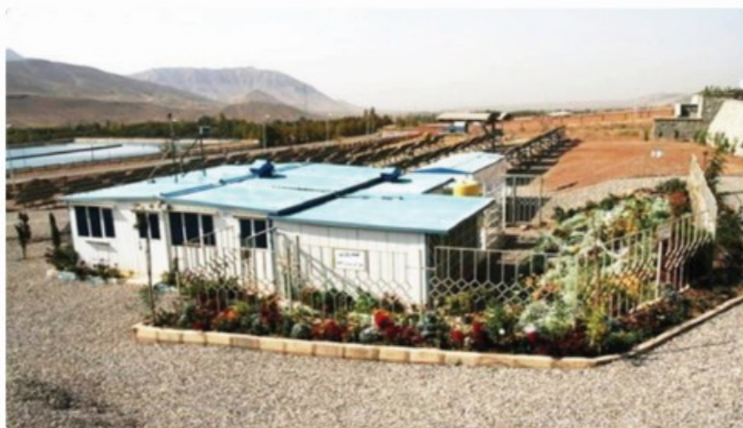
Taleghan Renewable Energy Park: Center for H 2 & FC technology demonstration and other types of renewable energy
